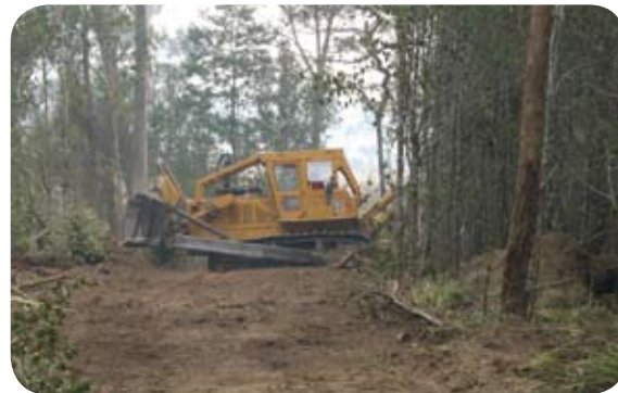
Earthmoving equipment is used during firefighting for construction of access roads and fire breaks. Photo courtesy of Paul Black, PWS.
